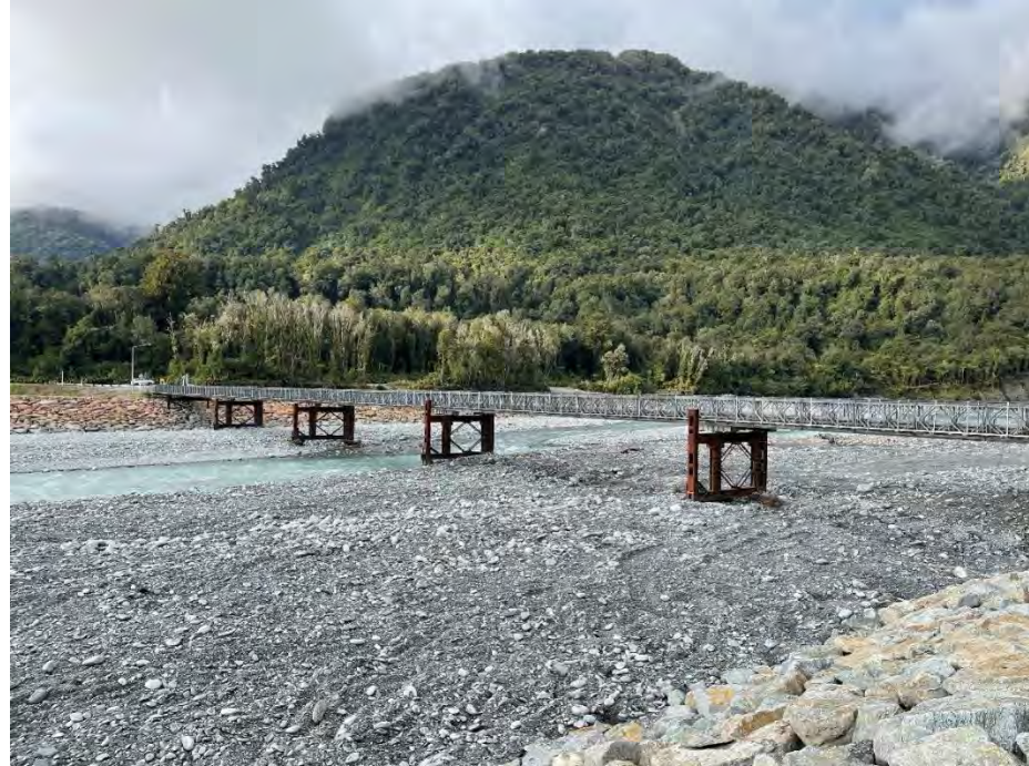
Figure 19. Waiho River Bridge south of Franz Josef
